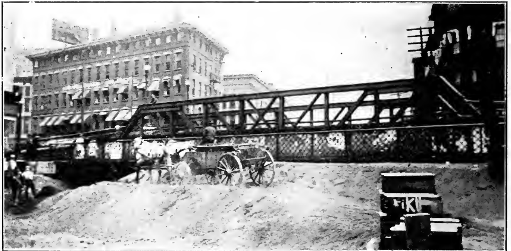
GRADING PREPARATORY TO REMOVING HIGHWAY BRIDGE WITHOUT INTERRUPTING TRAFFIC
